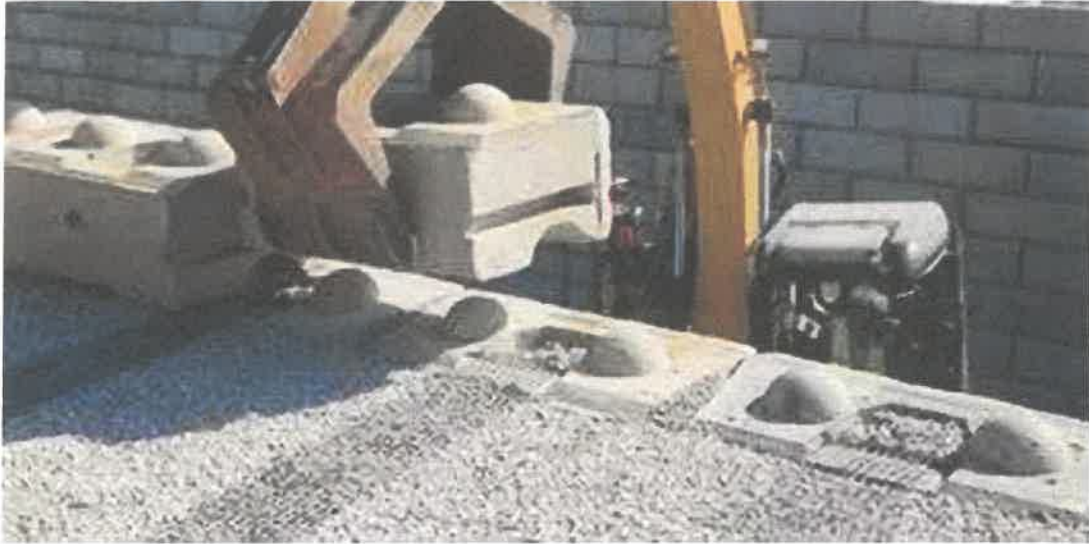
Example of placing Redi Rock block wall
