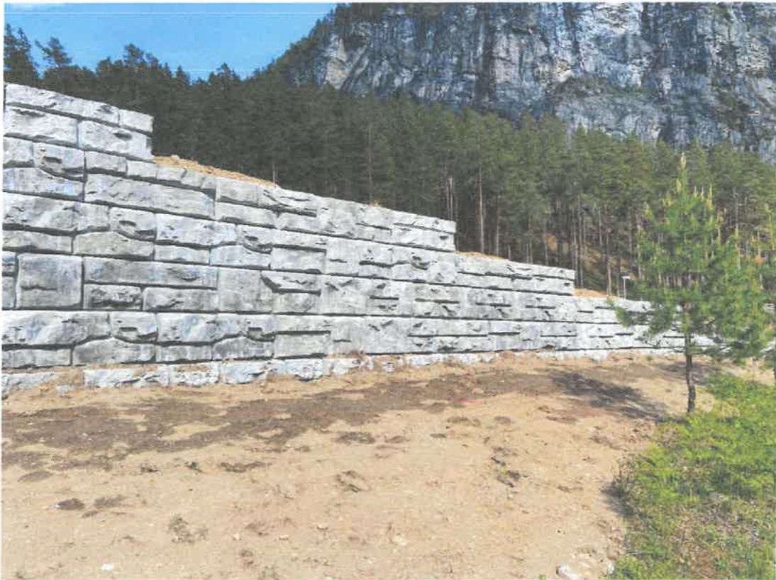
Example of Redi Rock block wall in alpine environment
